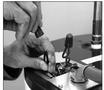
Figure 20 - Connecting the electrical wires. (Shroud not shown.)
