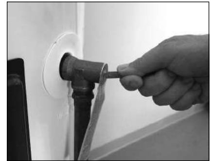
Figure 37 - T&P Relief Valve
