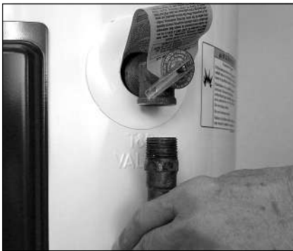
Figure 11 - Removing the T&P Relief Valve discharge pipe.
