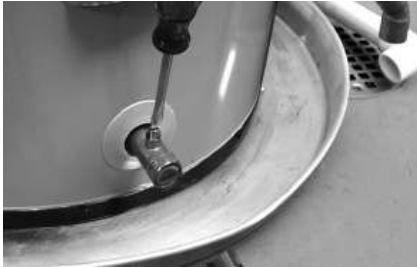
Figure 10 - Draining the old water heater.
